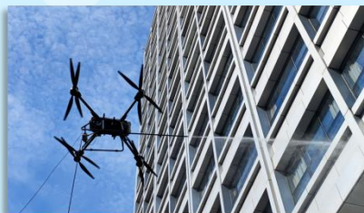
楼宇清洗 Building cleaning
