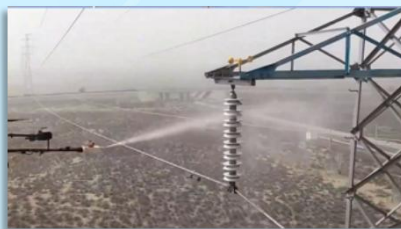
电网喷涂 Grid Spraying
